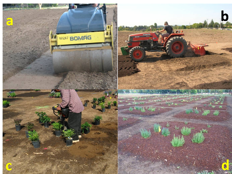
Figure 1. Field trial installation, Sept 2008. Soil compaction with vibrating roller (a), tillage treatment (b), plant installation with power auger in no-till treatment (c), all plots planted and mulched with Douglas-fir bark (d).
